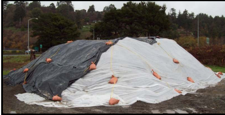
Proper securing of plastic sheeting.
