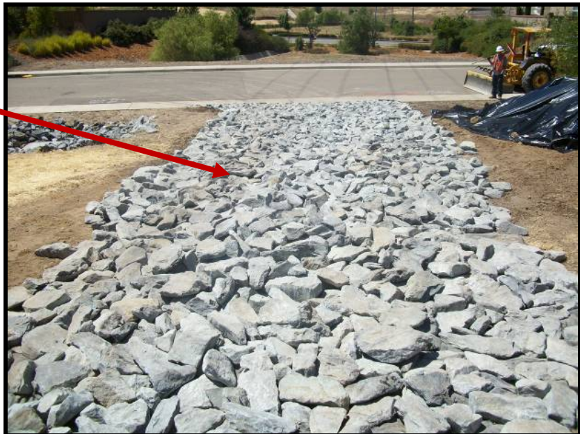
Traditional rocked construction entrance/exit.
