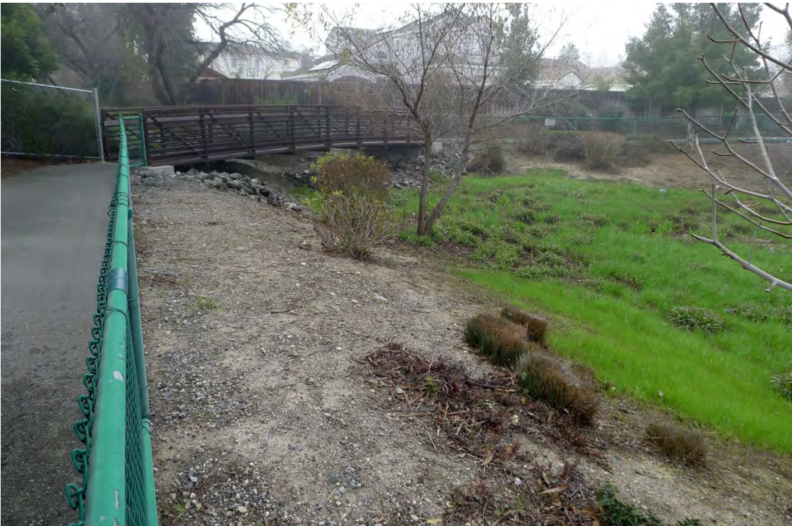
View of drainage inlet into detention basin from future outfall, looking S (1/21/15)
