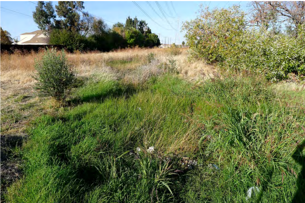
Surface drainage below culverts, looking N (11/17/14)
