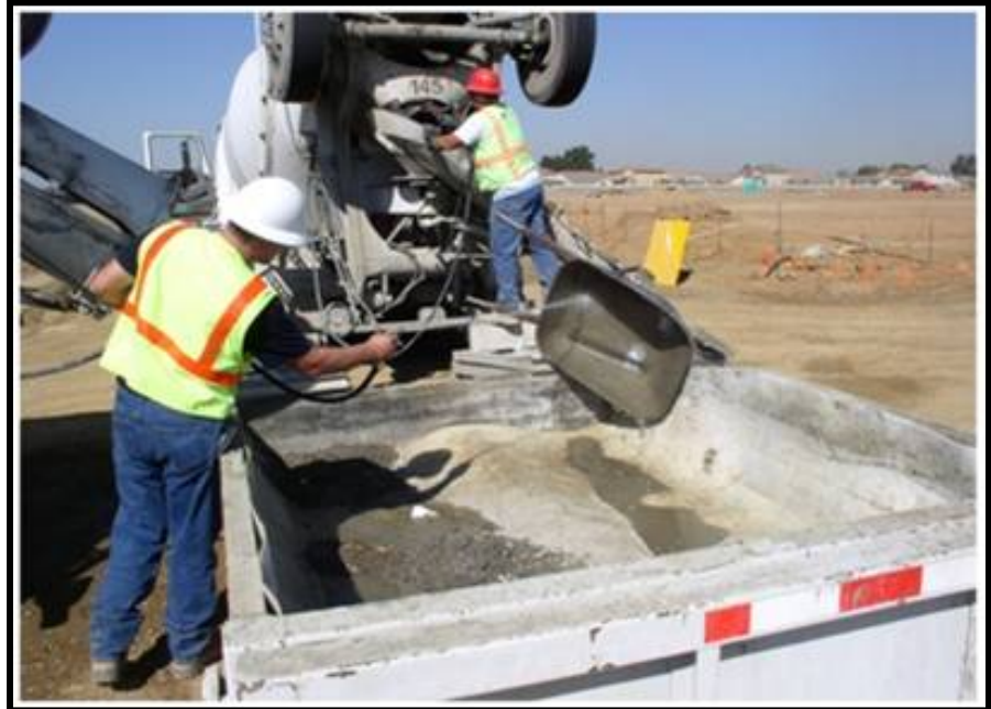
Self contained concrete washout.
