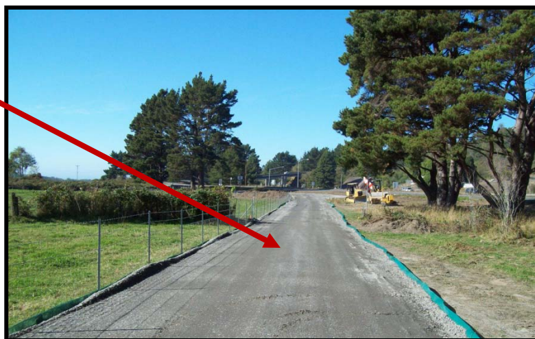
Stabilized construction road.
