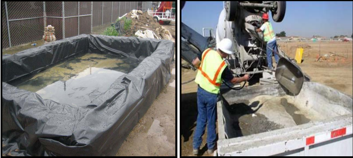
Two alternatives for containing concrete washout water.
