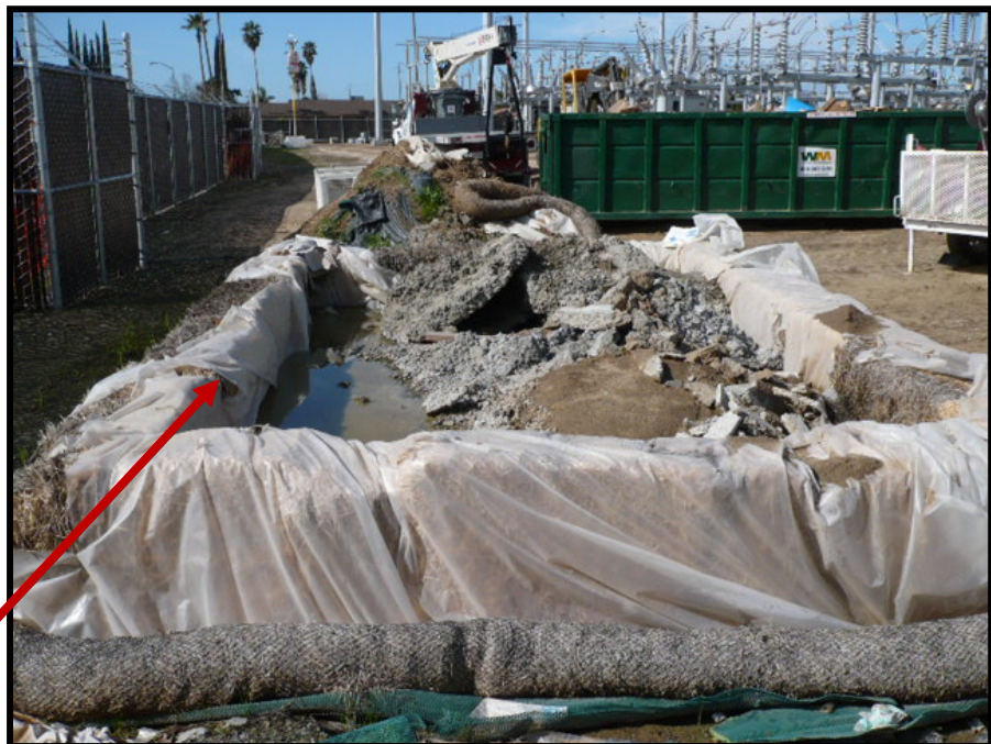
Lined concrete washout.
