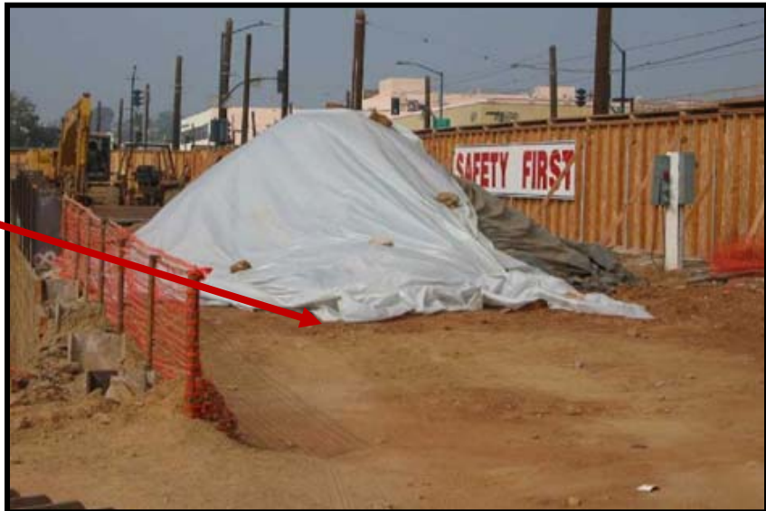
Stockpile covered with plastic and secured with large rocks. Where more than one sheet of covering is required, overlap sheets and secure at seam.
