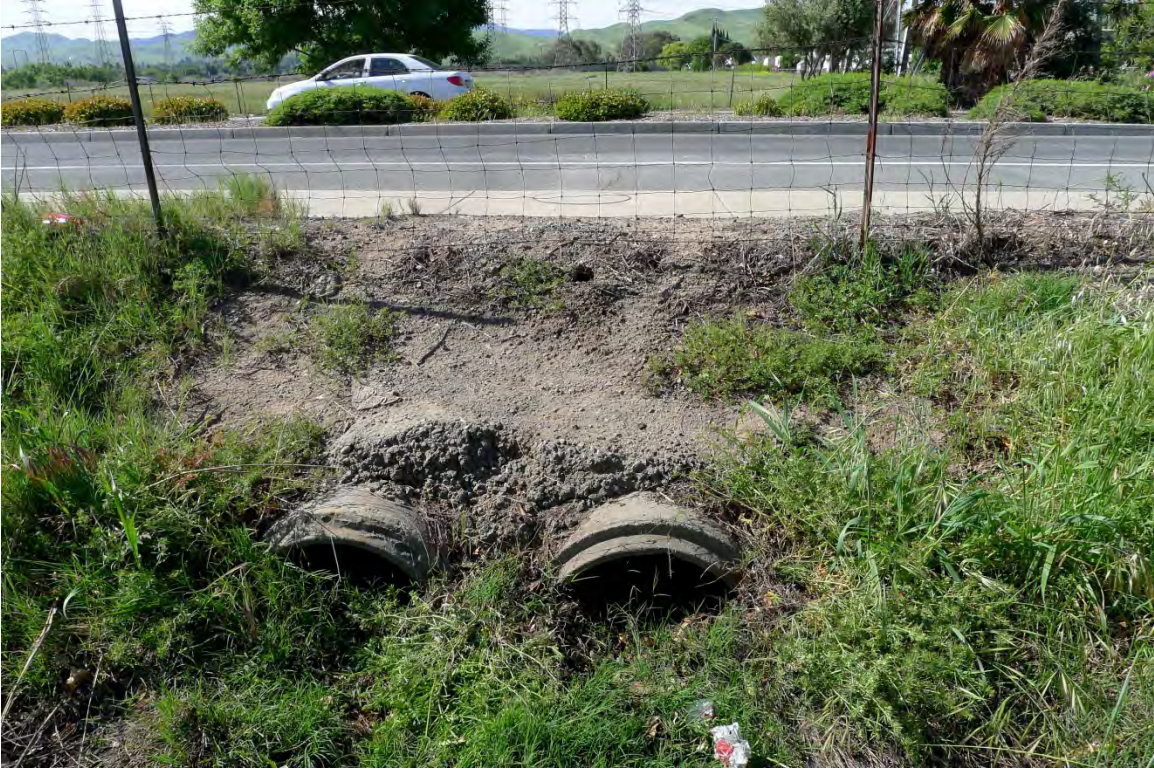
Culvert outfall at S end of study area, looking S (4/17/14)
