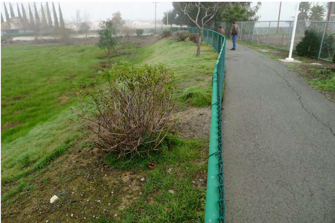
View of future basin outfall location, looking N (1/21/15)
