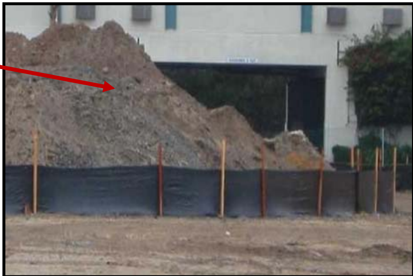
Silt fence as stockpile perimeter control.
