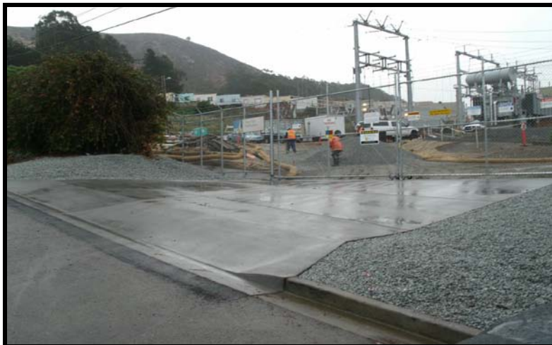
Clean and well maintained construction entrance/exit.
