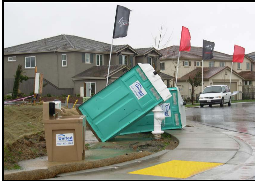
Locate sanitary facilities away from sensitive areas and secure to prevent overturning in high winds.
