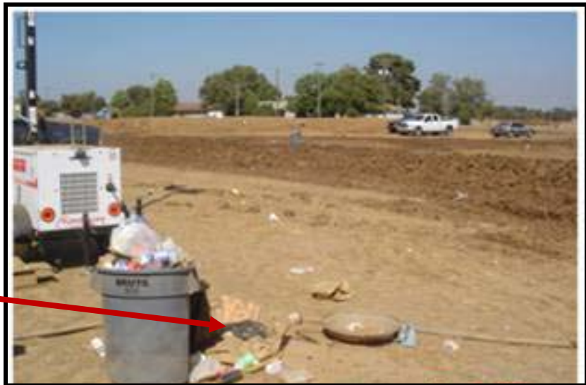
Improperly managed waste receptacle.
