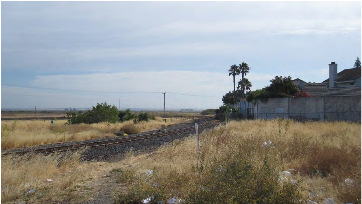
Photo 2: A 10-foot high concrete wall separates the railroad ROW from residence to the south. The wall blocks views of the parcel from neighborhoods to the south with exceptions for the second story of some two-story units.
