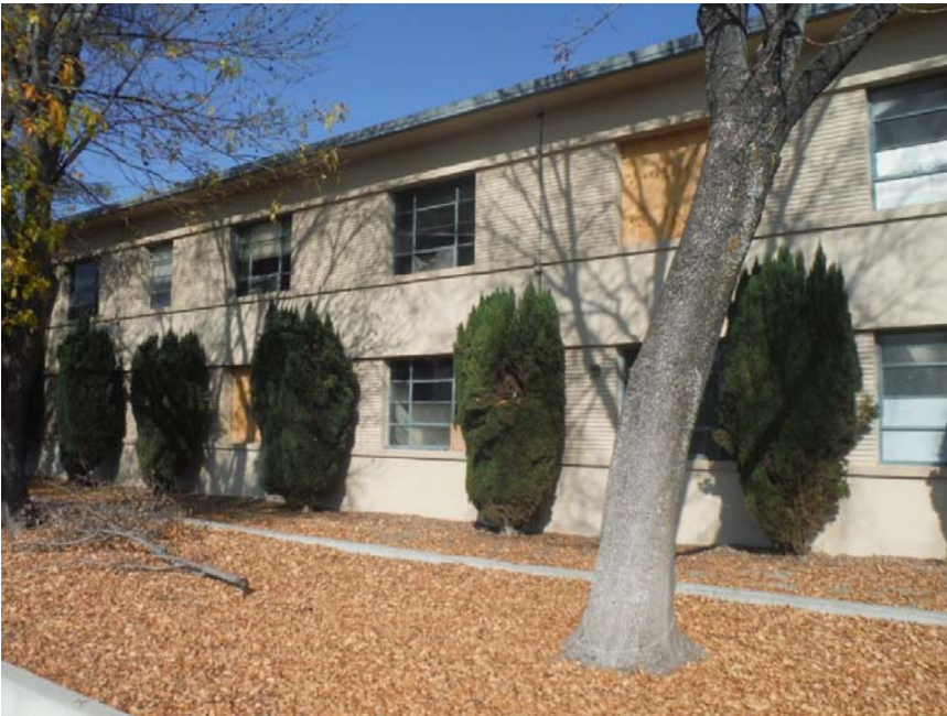
Photo 3: View northwest: Window detail on facade (west wing).
