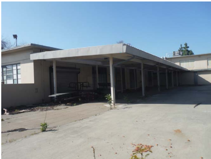
Photo 10: View southwest: Awning extending from rear of west wing (cafeteria). Recently installed roll-up door visible at left of photo. Patio covering former pool visible at right of photo.
