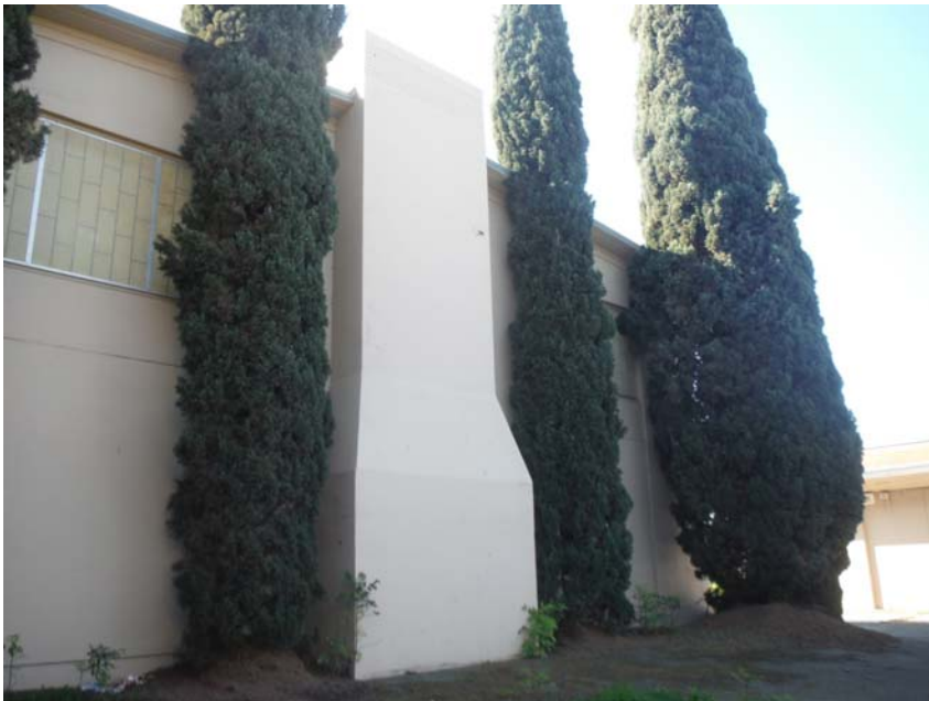
Photo 9: View southwest: Rear of library. Large external chimney and cypress trees visible.
