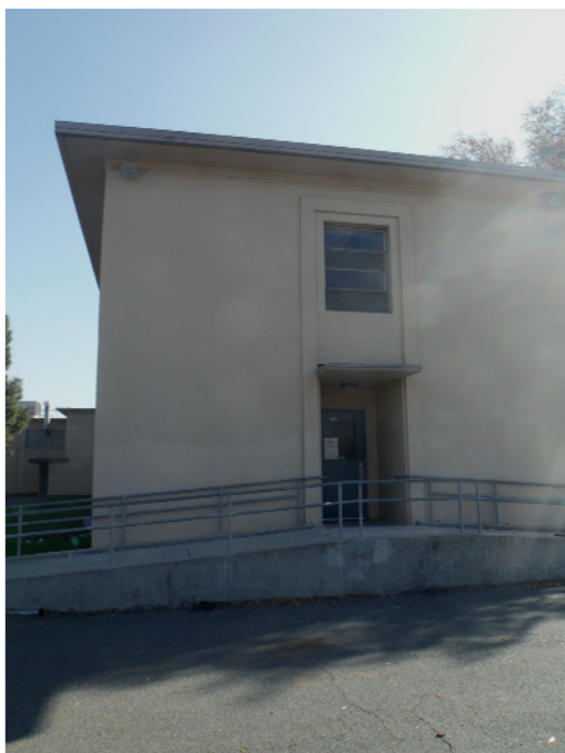
Photo 5: View southeast: West end of west wing with recently installed ADA compliant ramp. Representative flat awning over entrance is visible.
