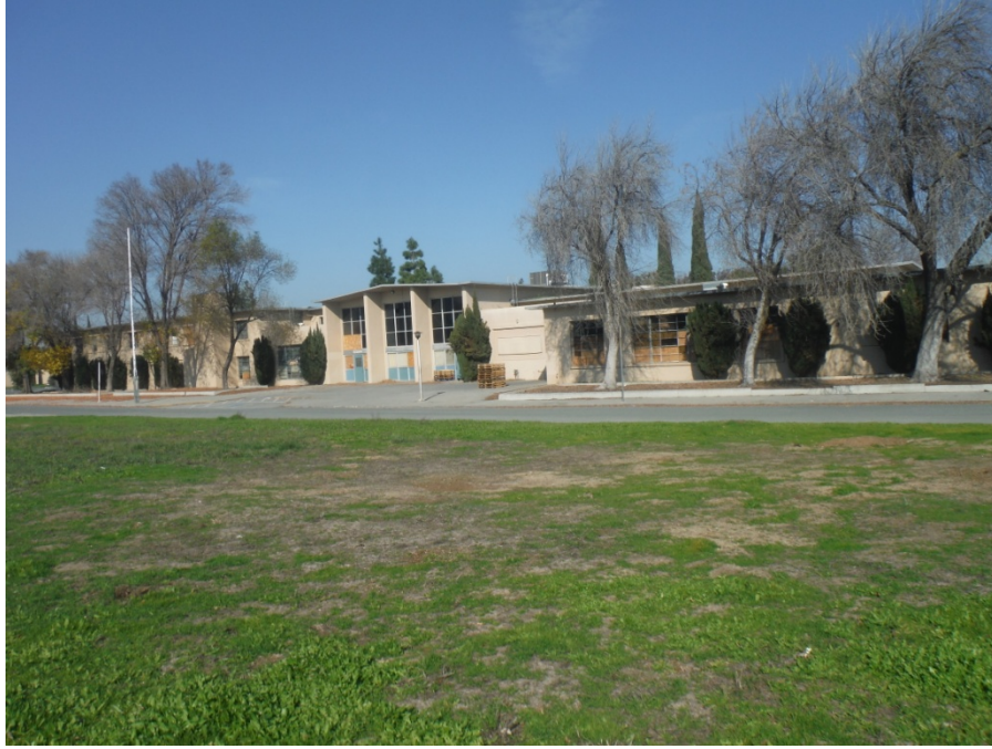
Photo 1: View northwest: Facade (south elevation) of former Officer's Club.
