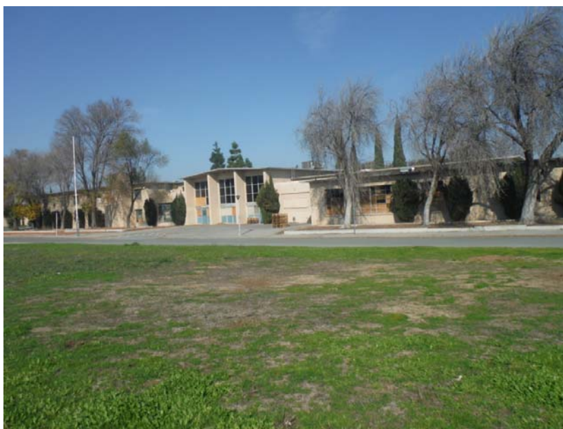
Photo 1: View northwest: Facade (south elevation) of former Officer's Club.
