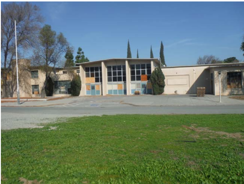
Photo 7: View north: Recently installed elevator likely visible at left of photo attached to front of building.
