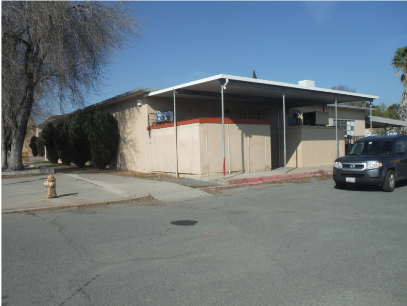
Photo 6: View northwest: Awning over utility equipment at east end of east wing.
