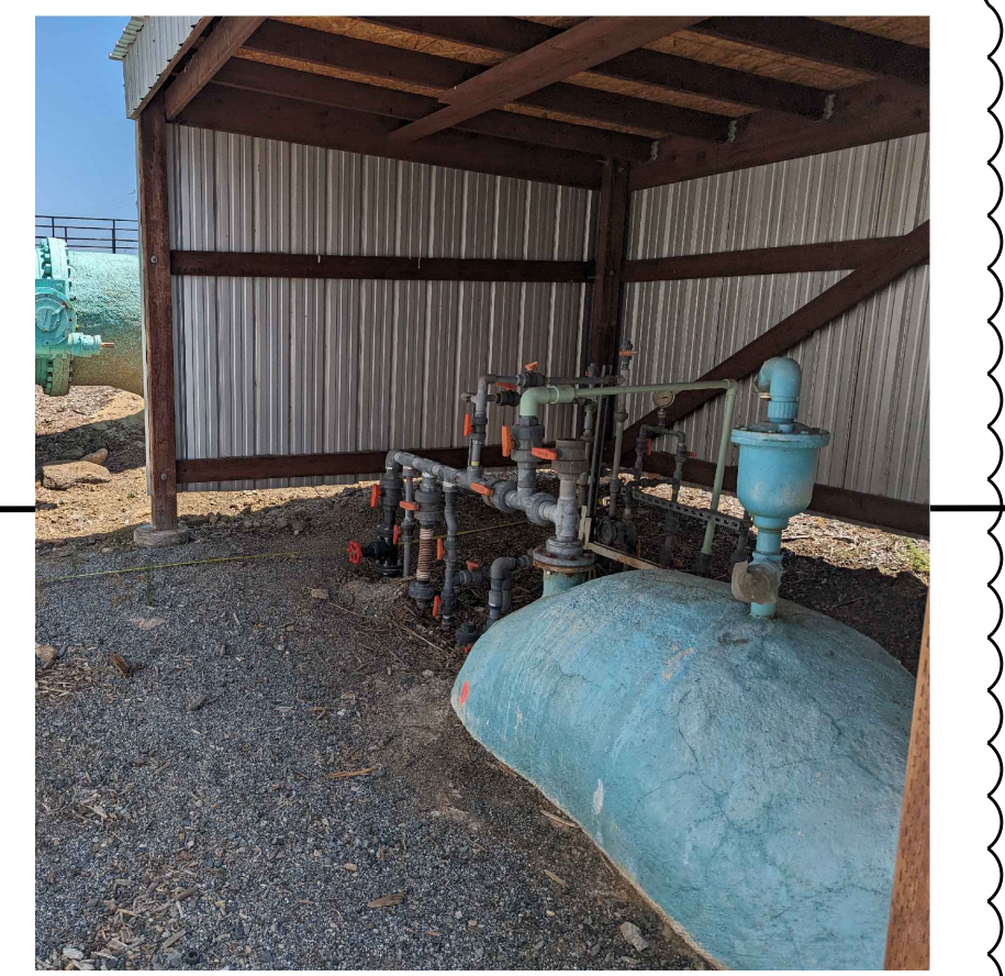
EXISTING INJECTOR BUILDING PHOTO 1
