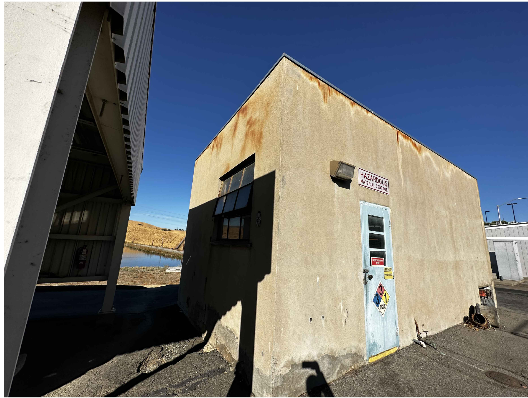
SE EXTERIOR OF BUILDING 43 PHOTO 1
