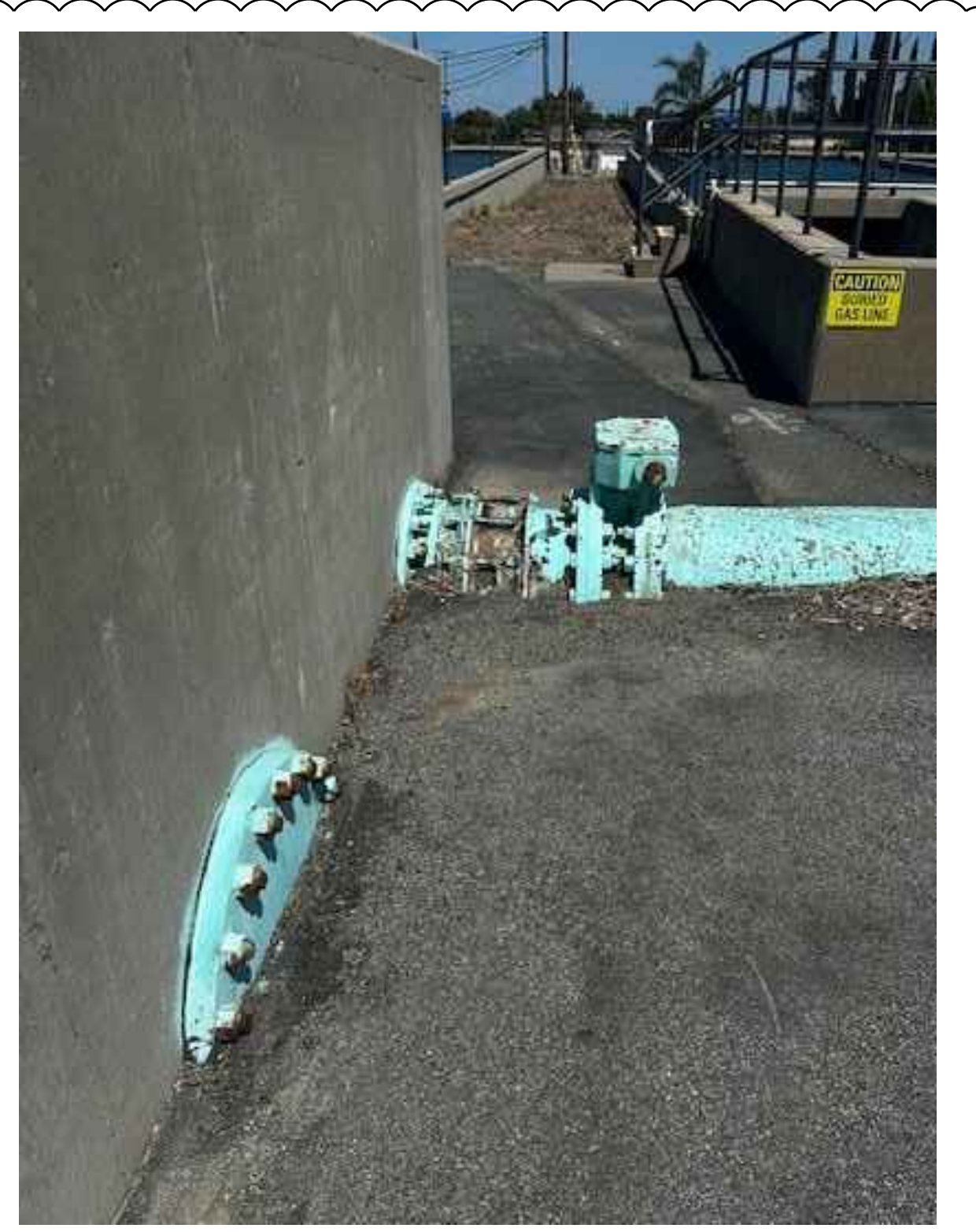
PICTURE 1 EXISTING 18" BFV (VIEW FROM EAST)
