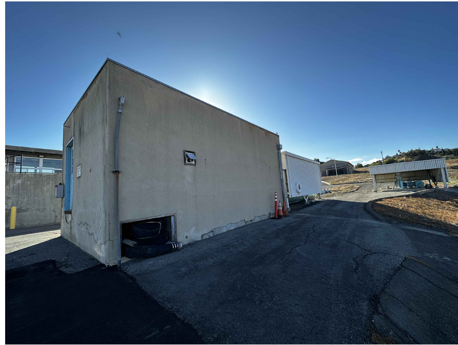
W EXTERIOR OF BUILDING 43 PHOTO 2
