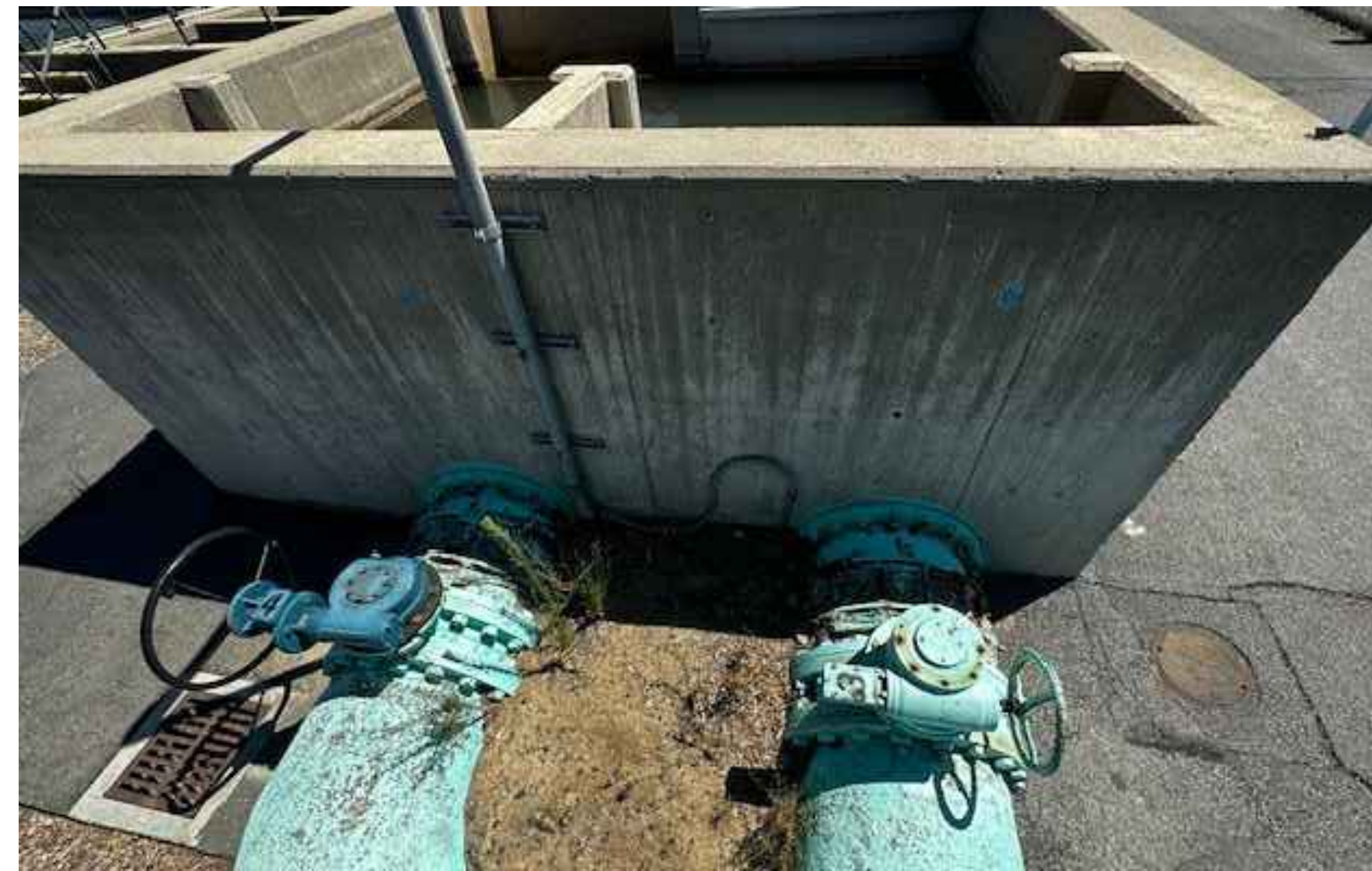
PICTURE 2 EXISTING 18" BFV'S (VIEW FROM TOP)
