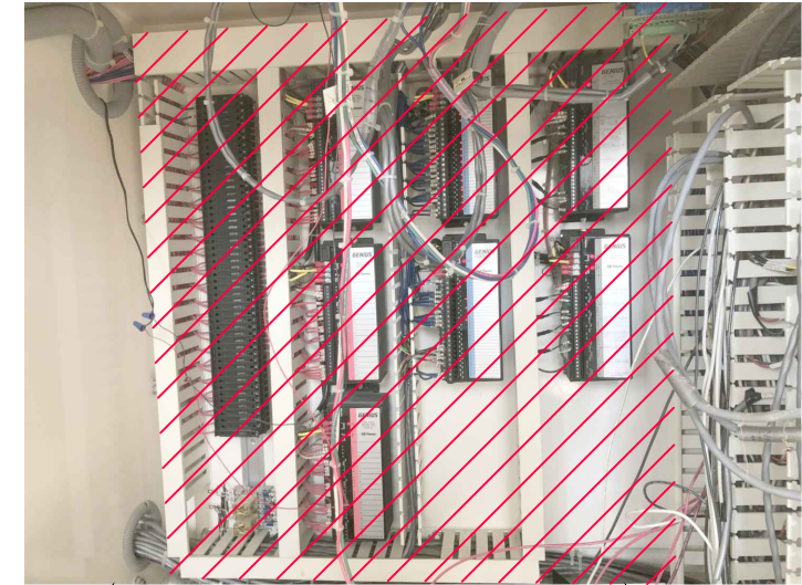
FILTER CONTROL CONSOLE 1/3, 2/4, AND 5/7 CONTROL PANEL (FCC 1/3, 2/4, 5/7) DEMOLITION
