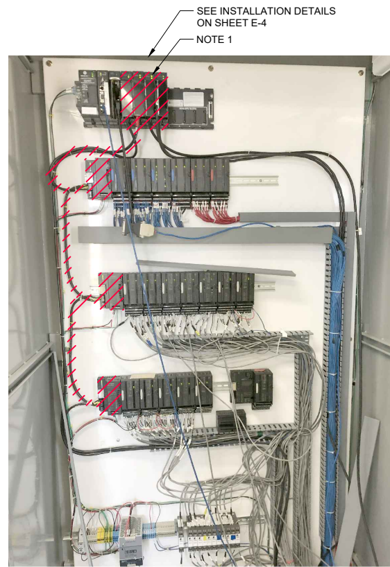
MAIN CONTROL PANEL (MCP) DEMOLITION
