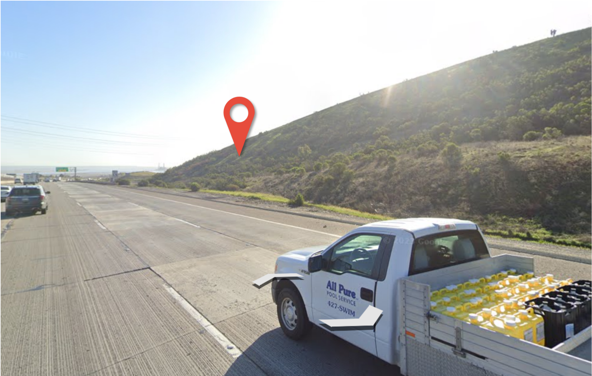
1: State Route 4 at Western City Limit
