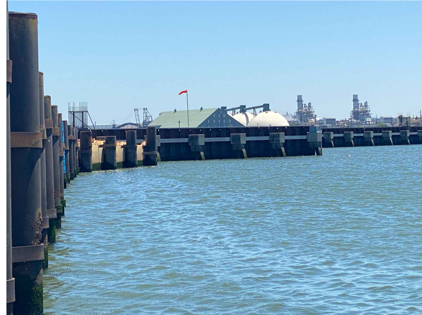
PHOTOGRAPH 2 BASIN 3 SHEET PILE WALL (DREDGE AREA A)
