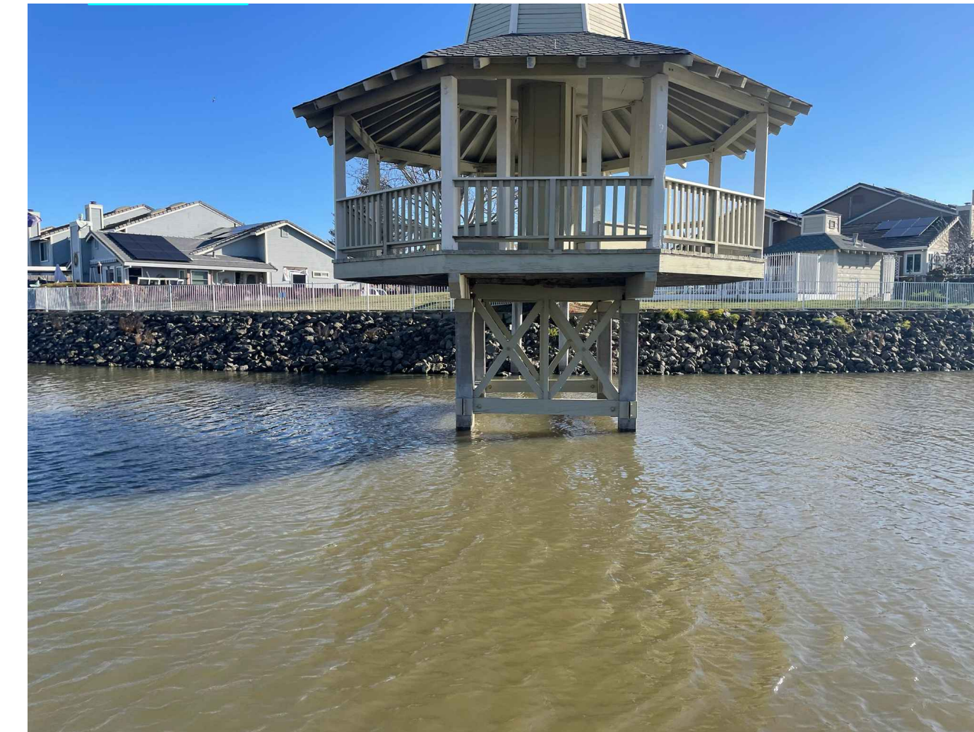
PHOTOGRAPH 6 RESIDENTIAL CHANNEL GAZEBO (DREDGE AREA C)
