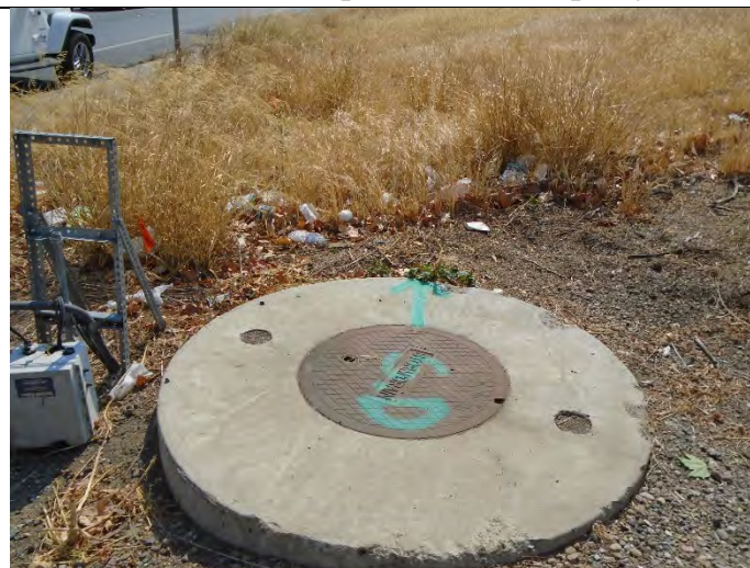
View East of onsite Storm Drain manhole in northwest portion of Property
