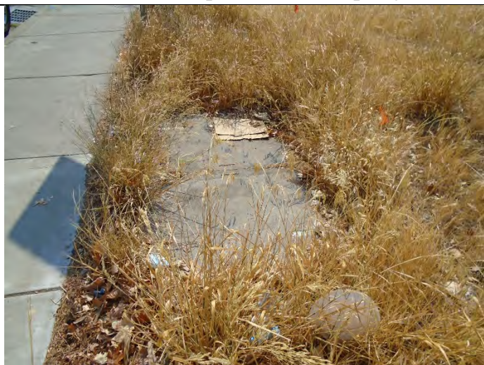
View East of onsite PG&E vault and electrical line easement in northwest portion of Property
