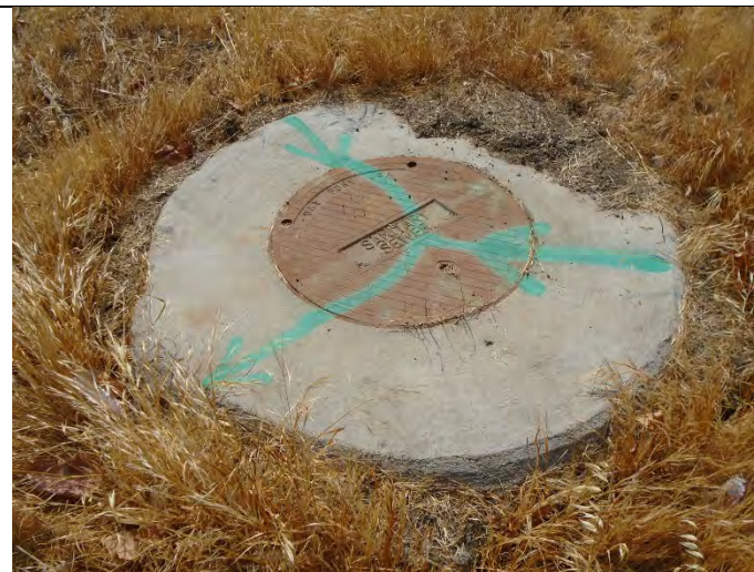
View North of onsite Sanitary Sewer manhole in northwest portion of Property
