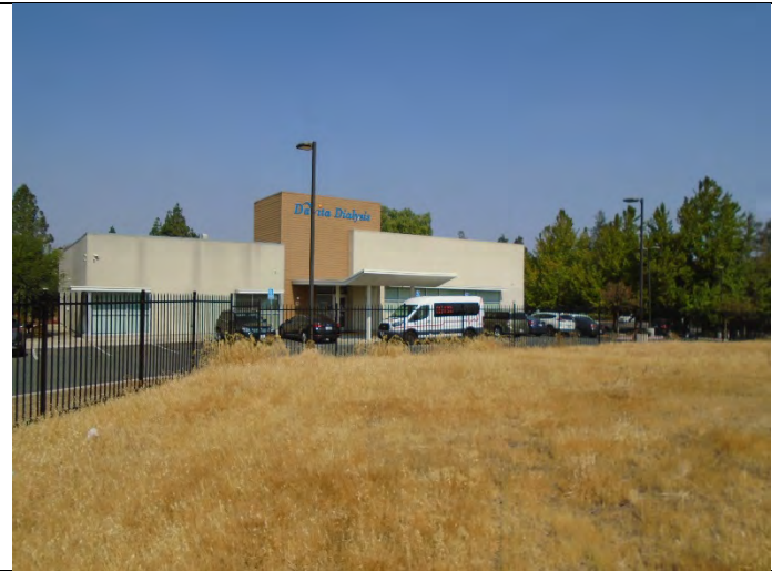
View West toward adjoining properties
