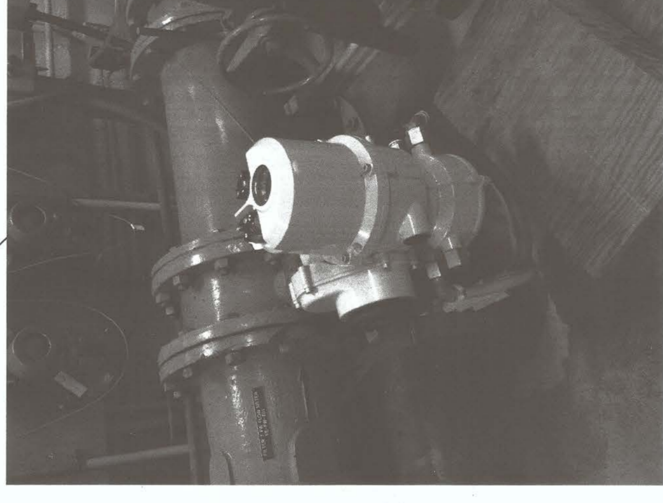
REPLACE VALVE-705 ELECTRIC ACTUATOR BFV-FW-705 TO REMAIN
