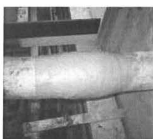
Wrapping and patching
