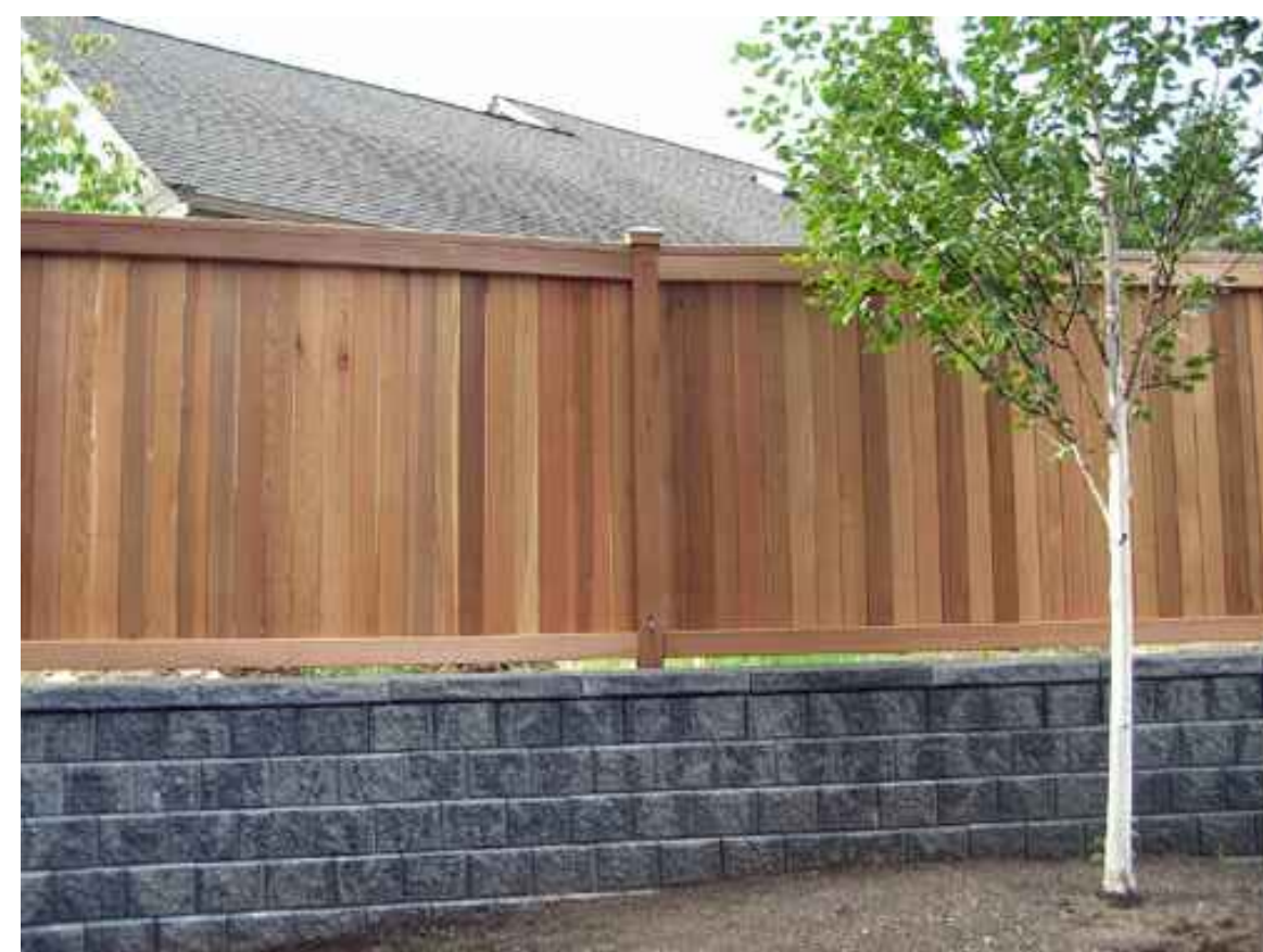
GOOD NEIGHBOR FENCE ON RETAINING WALL
