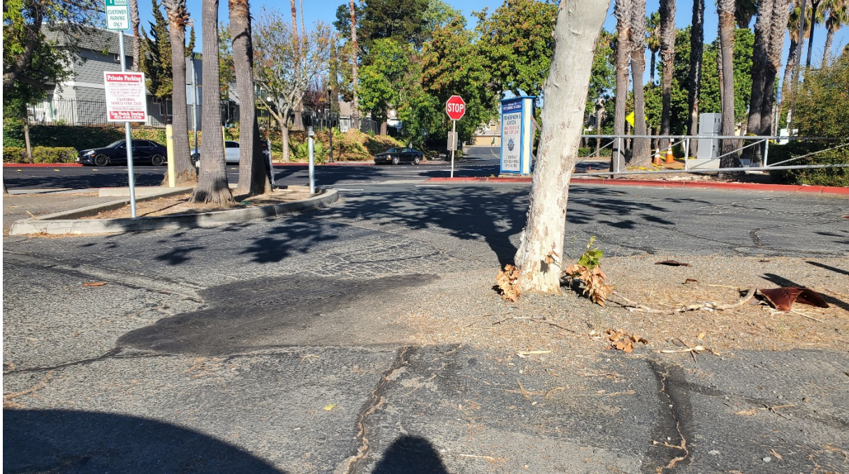
Site looking southwest
