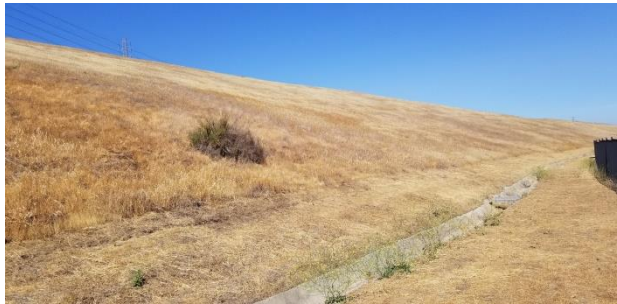
Figure 19.a – Point of view looking west
