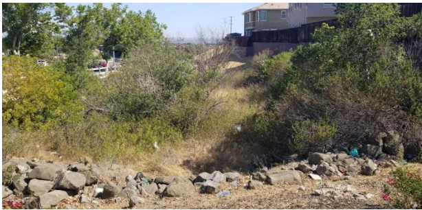
Figure 15.a – Point of view looking north
