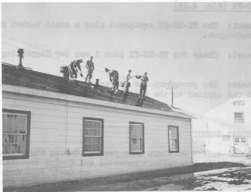
Fig. 2.11 Firehosing Roof Area. Procedure: On the first pass, the operator worked at a faster rate. Then the area was cleaned up firehosing was at the same rate as for the first procedure.
