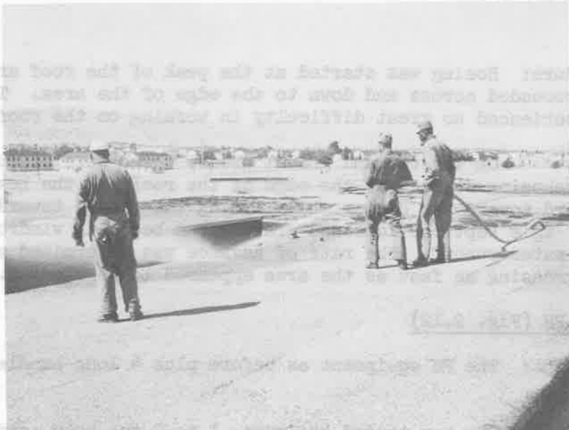
Fig. 2.11 Firehosing Roof Area. Procedure: On the first pass, the operator worked at a faster rate. Then the area was cleaned up firehosing was at the same rate as for the first procedure.
