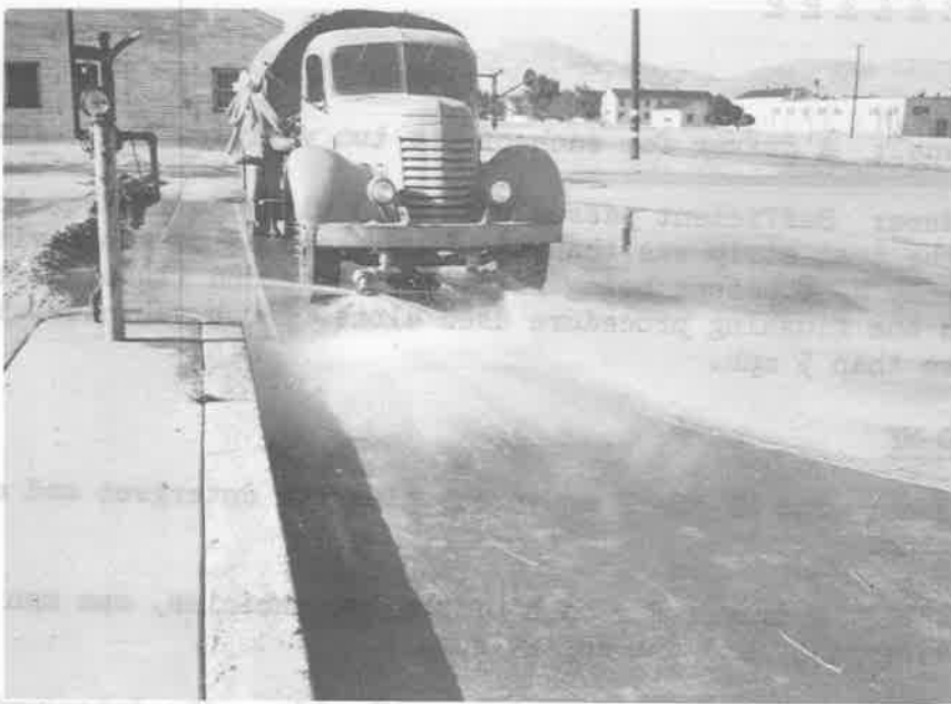
Fig. 2.9 Motorized Flushing Roadway
