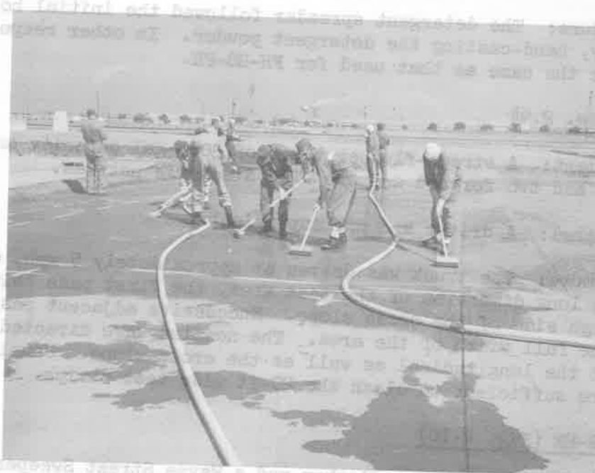
Fig. 2.8 Firehosing and Hand Scrubbing Paved Area.
