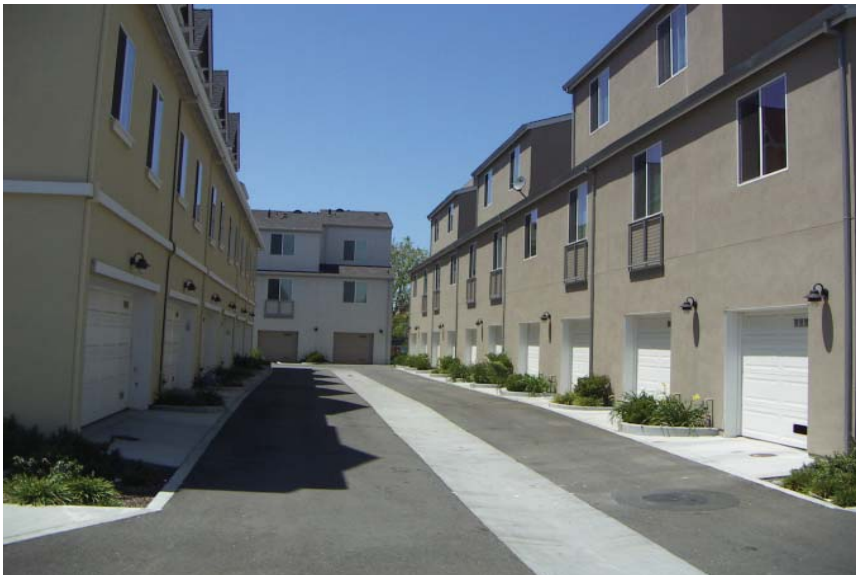
Alley-loaded garage doors are an alternative to garages that front on the public right-of-way.
